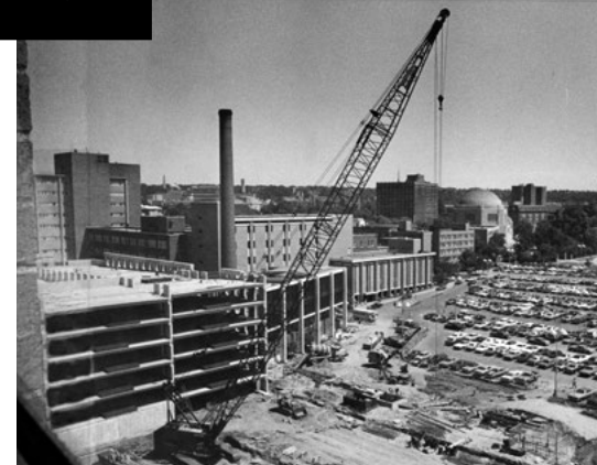
Mt. Sinai (Medical Center) construction, 1973
