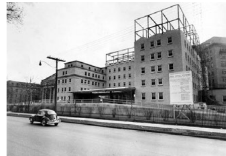
Metropolitan General Hospital construction, circa 1962 Image: courtesy of the Michael Schwartz Library Special Collections, Cleveland State University
